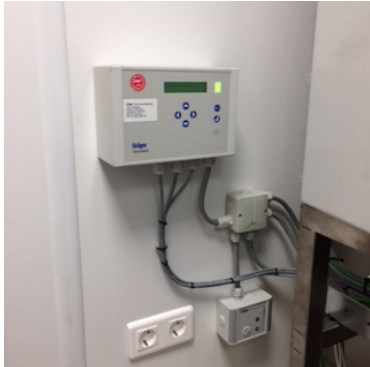
Figure 3 - Gas detection system
