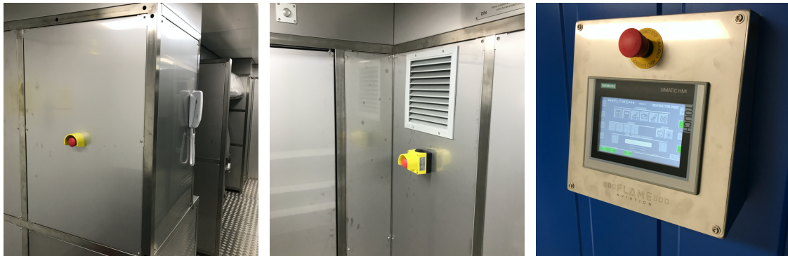
Figure 2 - Emergency stop buttons
