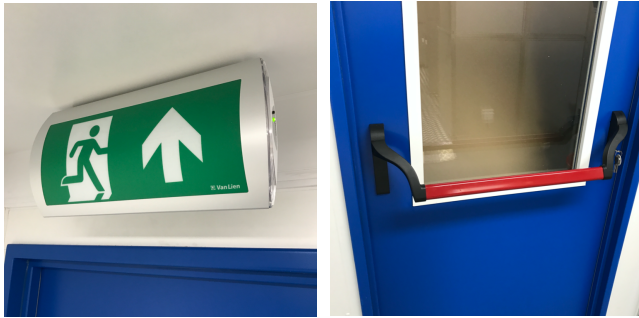
Figure 4 - Exit signs and panic escape handles
