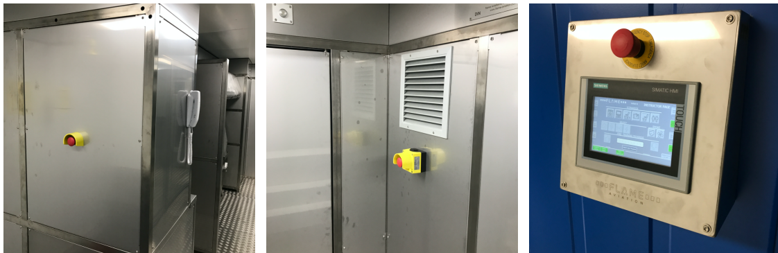
Figure 20 - Emergency stop button locations
