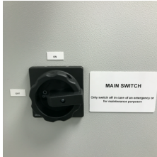
Figure 6 – Main power switch
