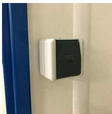
Figure 8 – Light/standby switch
