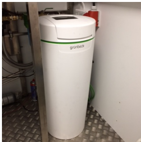
Figure 19 - Water de-calcifier unit
