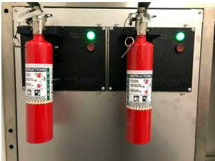
When the refilling process is finished, the green light will illuminate steady and the extinguisher will be released. The entire process shall not take more than 25 seconds.
