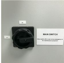
The fire trainer Main Power Switch in the Technical Room shall be ON.
