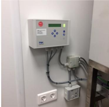
*Figure 3 - Gas detection system*
