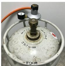
The gas bottle, normally located in the gas cabinet in the technical room, shall be opened by turning counter clockwise.
