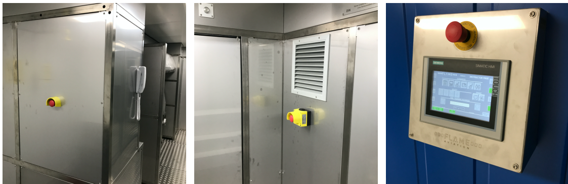
Figure 1 - Emergency stop button locations
